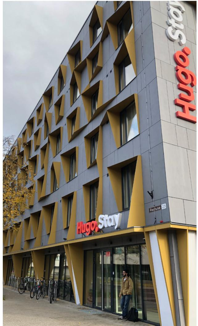
*"Since the construction time of the façade was during a cold and relatively wet winter period, building the elements in factory conditions made a lot of sense from a quality perspective. Besides the quality control benefits the offsite approach allowed us to minimize and control the actual site time by getting the box insulated and weatherproof as fast as possible and start with interior work. Our site crew was very satisfied with the overall solution"*
